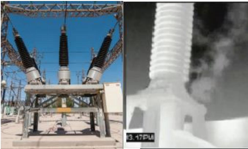
Caption: Detecting invisible SF<sub>6</sub> leaks from circuit breakers
