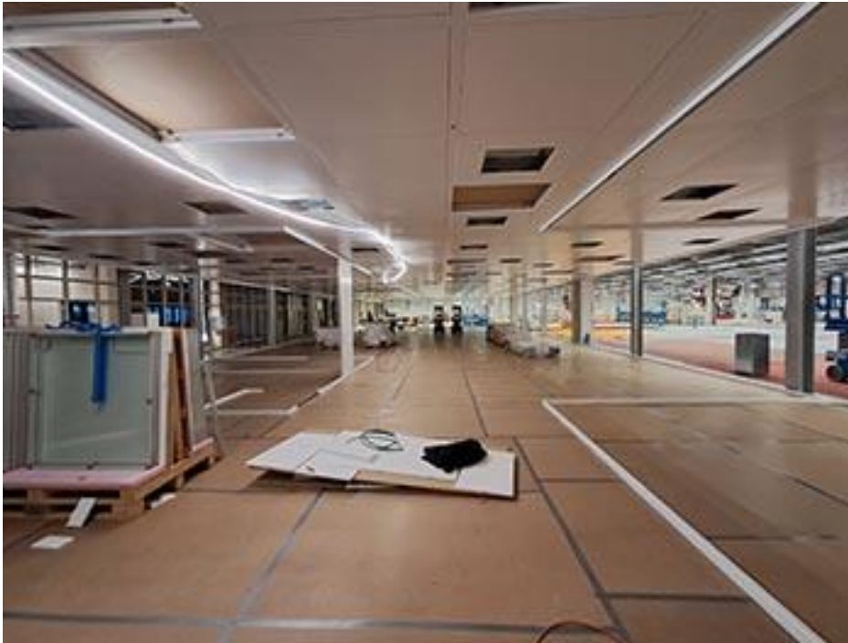
Caption Picture 3 and 4: Installation of the cleanroom walls
