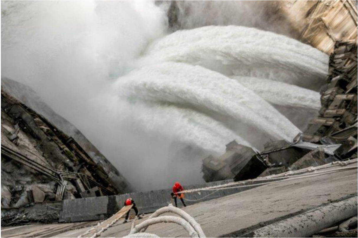
The Wudongde Dam from above
